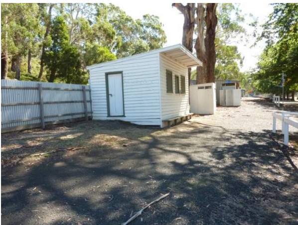
Various race club buildings, west of track
