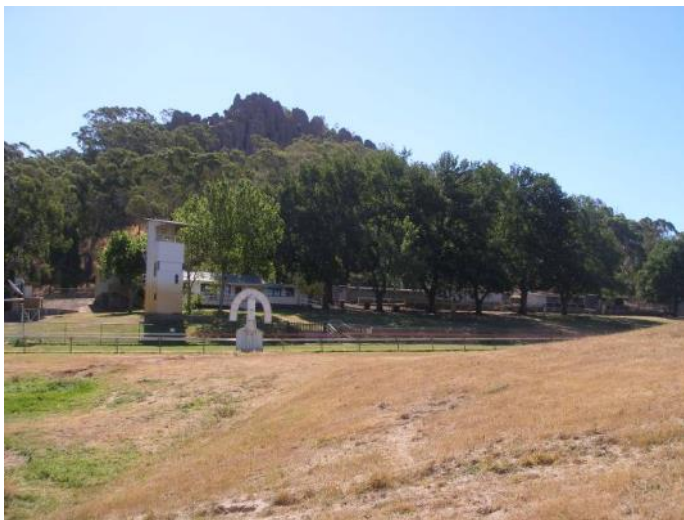
Figure 10. View back to Hanging Rock above the racecourse building complex from the dam end of the reservoir.
